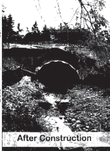
Figure 18. The new crossing is a corrugated aluminum arch culvert, 3.8 meters (12-foot) wide, with natural stream-bed material to simulate a natural condition throughout the culvert. This fish passage project restored access to 2.4 kilometers (1.5 miles) of potential habitat for coho salmon, and steelhead, searun and resident cutthroat trout.
