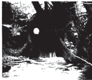
Figure 5. The old culvert was a round concrete pipe, 1.83 meters (6-foot) diameter. The culvert was assessed as a fish passage barrier due to a 0.50 meters (1.64-foot) water surface drop and a 2.5% slope.
