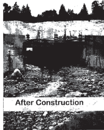
Figure 20. The new crossing is a concrete box structure, 3.8 meters (12-foot) wide with natural streambed material placed inside to simulate natural stream conditions throughout the culvert. This fish passage project restored access to 2.4 kilometers (1.5 miles) of potential habitat for coho salmon, and steelhead, searun and resident cutthroat trout.
