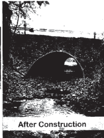
Figure 12. The new crossing is a round corrugated aluminum pipe, 3.05 meters (10-foot) wide with a streambed material placed inside the culvert to simulate natural stream conditions. This fish passage project restored 1.2 kilometers (0.75 miles) of potential habitat for chum, Chinook, and coho salmon, and steelhead, searun and resident cut-throat trout.
