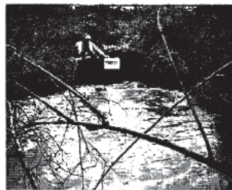
Figure 9. The old culvert was a squash corrugated steel pipe, 1.77 meters (5.8-foot) wide. The culvert was assessed as a velocity barrier.
