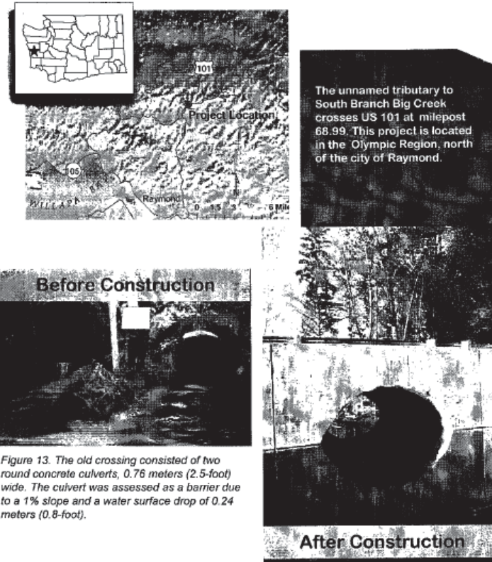
Figure 14. The new crossing is a corrugated aluminum arch structure, 5.5 meters (18-foot) wide with natural streambed material placed throughout the culvert. This fish passage project restored access to 4.6 kilometers (2.9 miles) of potential habitat for coho salmon, and steelhead, searun and resident cutthroat trout.
