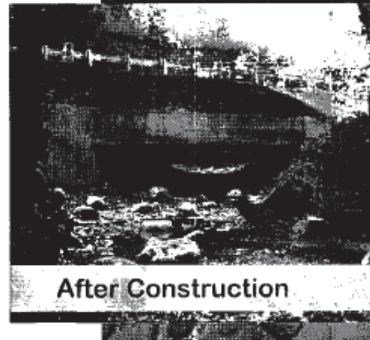
Figure 6. In the summer of 2011, WSDOT replaced the barrier culvert with a 7.62 meters (25-foot) concrete box culvert with natural streambed material. This fish passage project restored access to 11.3 kilometers (7 miles) of potential habitat for coho salmon, and steelhead and searun and resident cutthroat trout.
