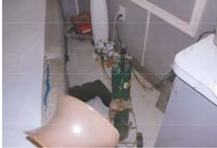
Procedure room, depicting ripped procedure table & stirrup, dust-covered oxygen tank, corroded tubing,
